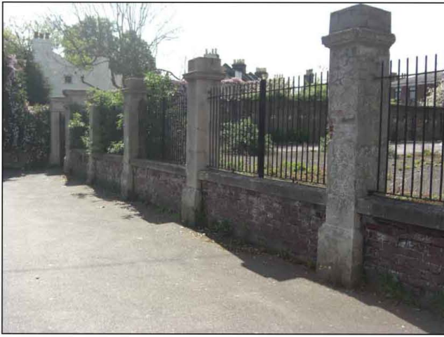
Plate 3. Original brick wall, rendered piers and railings. Facing south east.
