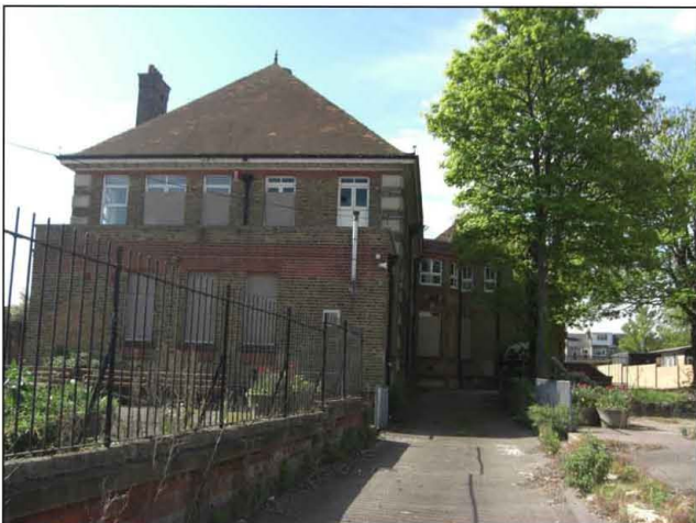
Plate 7. Entrance to western side of school bounded by brick wall and railings. Facing south.
