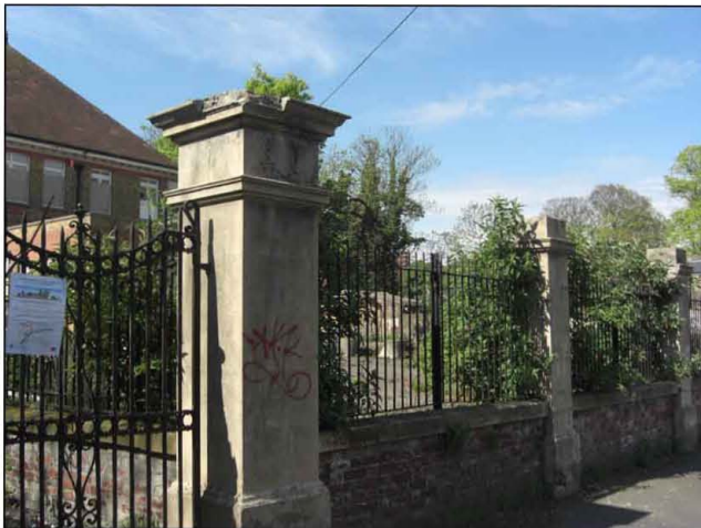
Plate 5. Decorated imitation stone piers. Facing south west.
